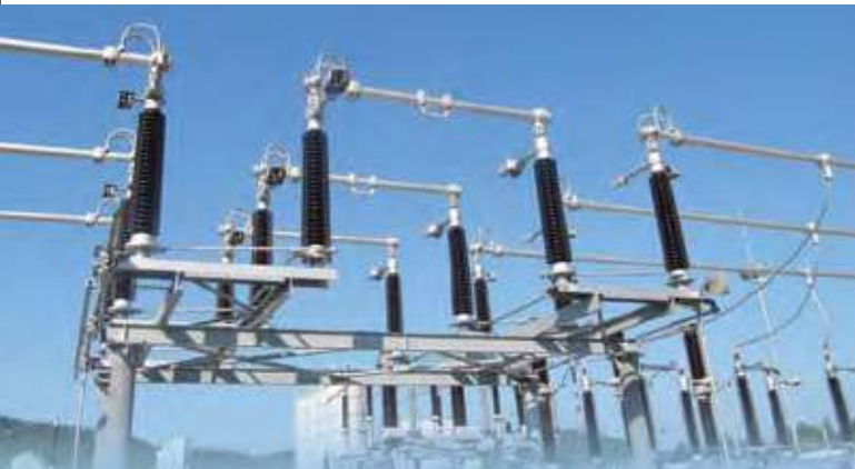
Centre Break Disconnector with Earth Switch
